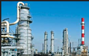
Oil & Gas Recovery
